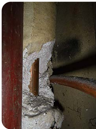
(Left) Asbestos-containing pipe lagging; and (Right) asbestos-containing gutters, capping and roof.
