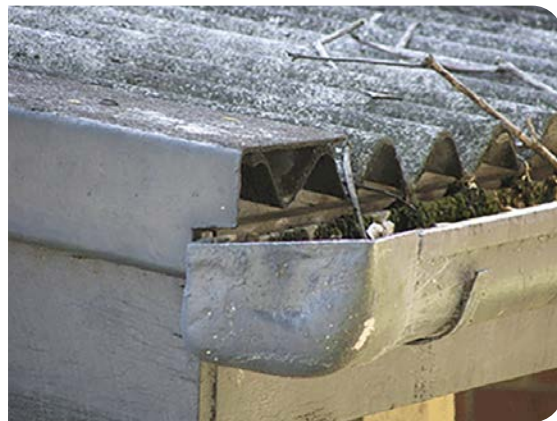
(Left) Asbestos-containing pipe lagging; and (Right) asbestos-containing gutters, capping and roof.
