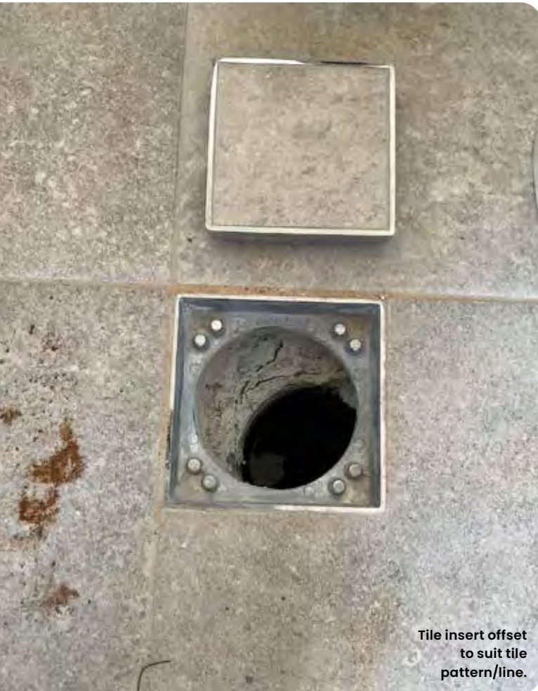
A combination of tile screed and tile adhesive presents a surface area that will be hard to clean, and more than likely encourage odours through the build-up of dampness and shower 'crud'.
